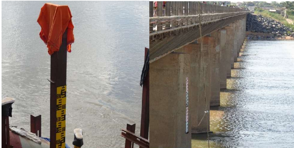
Figure 5. The ARA-Norte river gauges in use in Nante (left) and Mocuba city (right) in the LRB.
